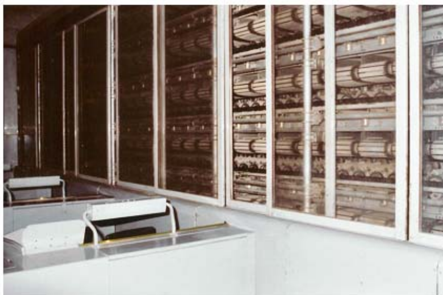
Figure 4 – A second view of the console area of the BTMC machine at Cairo from the opposite direction. This shows a rather clearer view of the sorting machinery.
