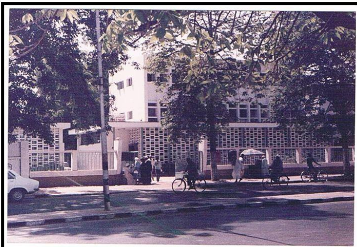
Fig.3. Aswan main post office, 1989
