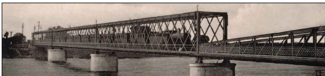
The completed bridge of 1895
