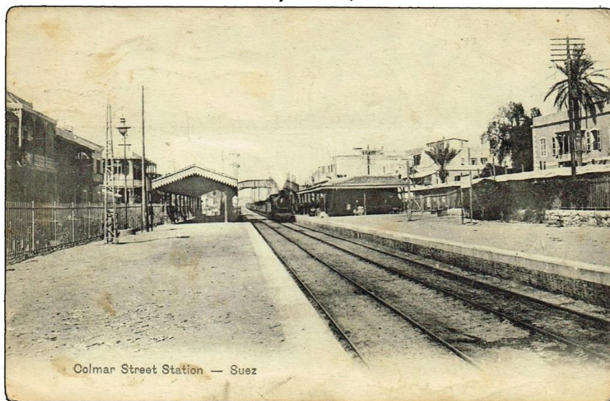
Colmar Street Station - Suez (C.A.)
