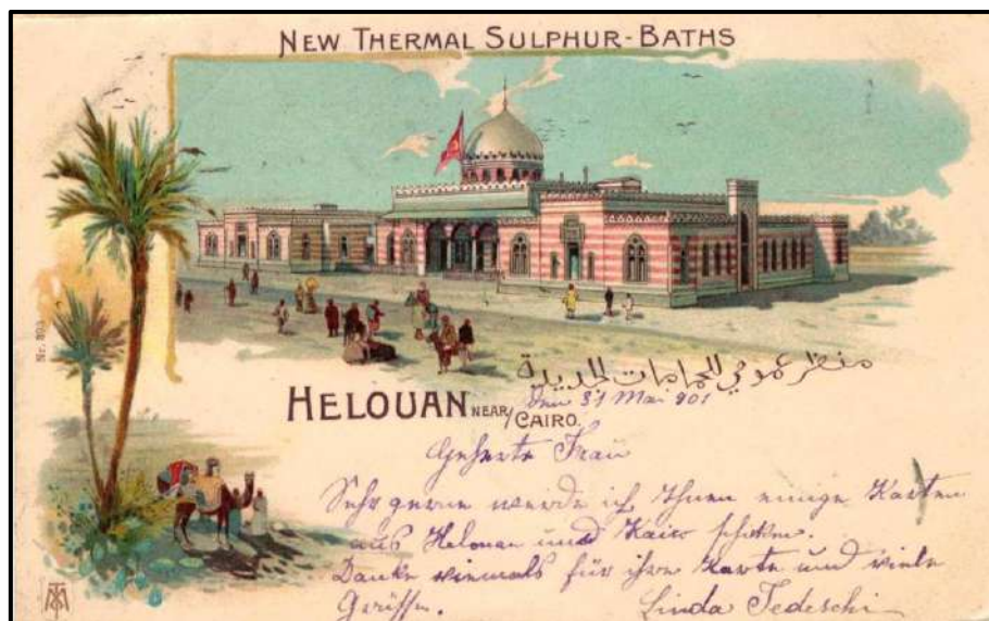
The single-storey New Thermal Sulphur Baths, addressed to Germany on 31 May 1901
